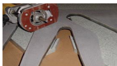
(8) Rout out cracked build up
