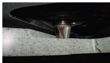
(4) Rout bevel into counter
